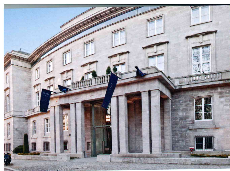
Clockwise from top left: The only modification to the landmarked 1940 limestone facade is a glassed-in entry. Custom-printed cotton covers part of the ceiling in reception, where seating is by Studio Urquiola. A guest suite's built-in headboard is cerused oak. The lobby features a bronze crocodile sculpture by Quentin Garel. The lobby features a bronze crocodile sculpture by Quentin Garel. A Studio Urquiola sofa in the lounge is strewn with pillows covered in wool-nylon.
